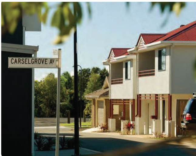
5.17 - Palmerston Laneway off Carselgrove Avenue (Fitzgibbon Chase)
