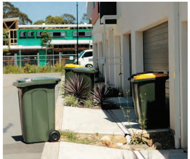
Figure 5.22 - Inadequate on-site bin storage leads to bins being left in the laneway. Dedicated accessible, screened, and ventilated bin areas should be provided in each lot and not in the garage.
