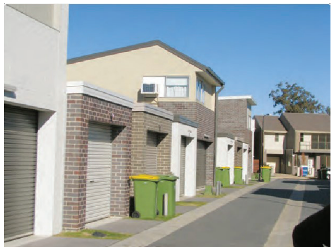
Figure 5.2 - Rear laneway with primarily access to garages
