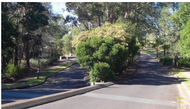
Figure 2.4 - Narrowing the pavement in short sections - Examples
