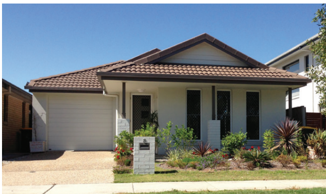
Figure 3.1 - Well-presented 3-bedroom cottage on small frontage lot
